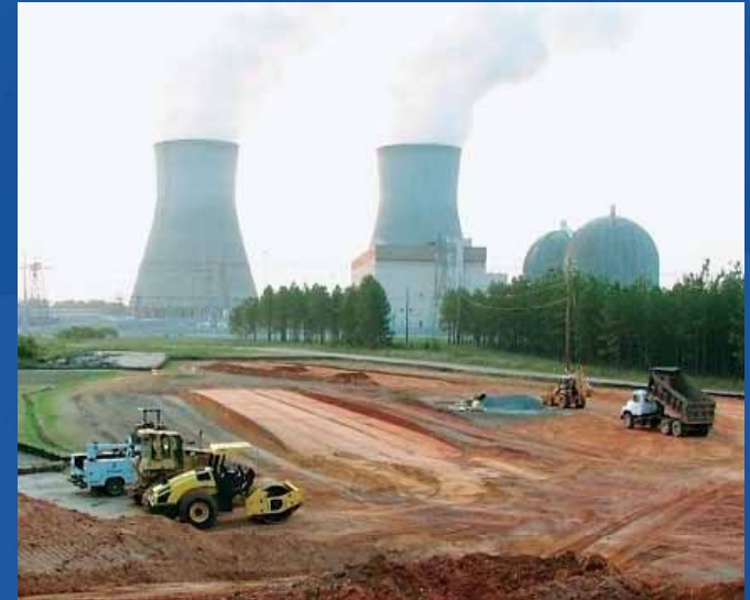
Vogtle site preparation
