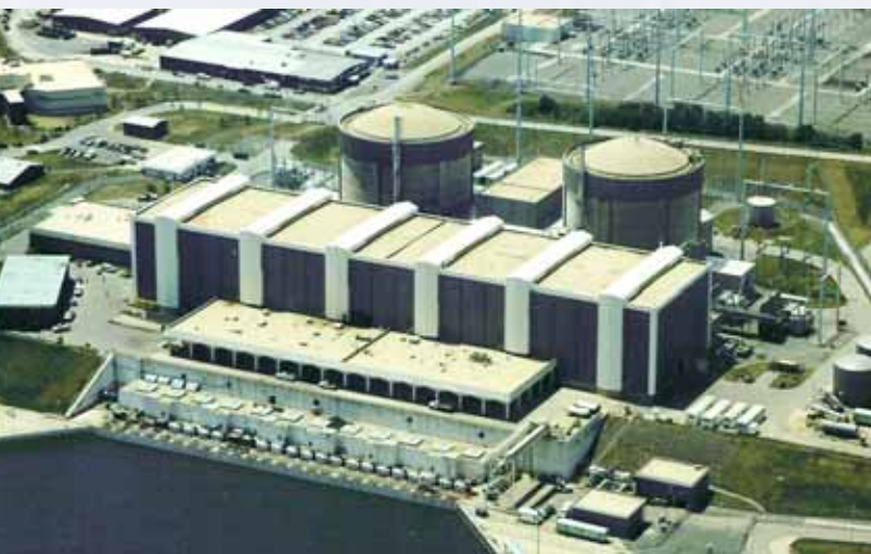
Calvert Cliffs Nuclear Power Plant
