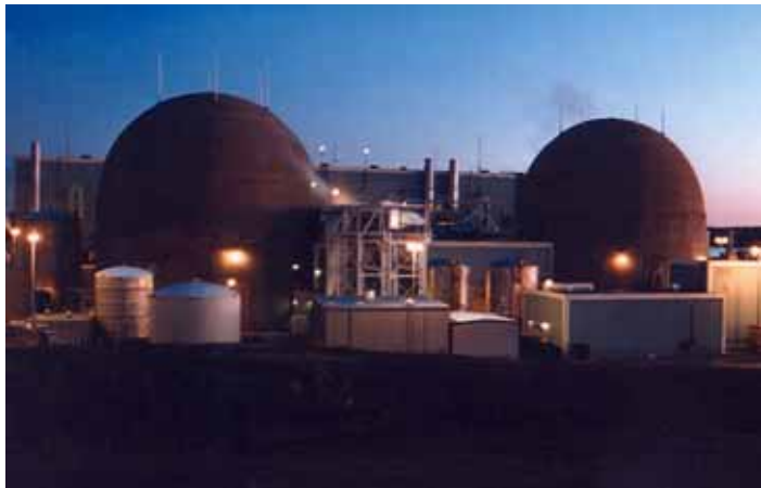
North Anna Containment Building
